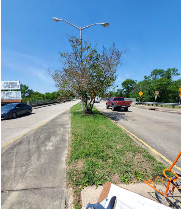
Before view of median
