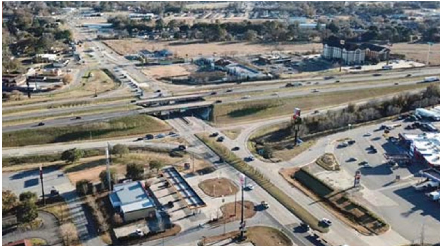
I-10 Ingress/Egress Ramps image from University Gateway report
