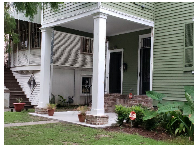
Porch floor removed and lowered to grade is an inappropriate alteration.
