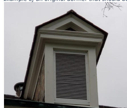
Replacing a dormer window with a louvers is an unacceptable change.
