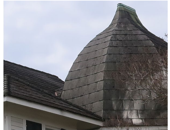
Asbestos roofs require special consideration when removed.
