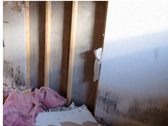
PHOTO: Remove all wet or fire-damaged insulation, even if wallboard appears to have dried.
