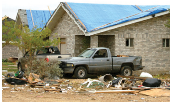
PHOTO: FEMA-provided "blue tarp" temporary roof protection.
