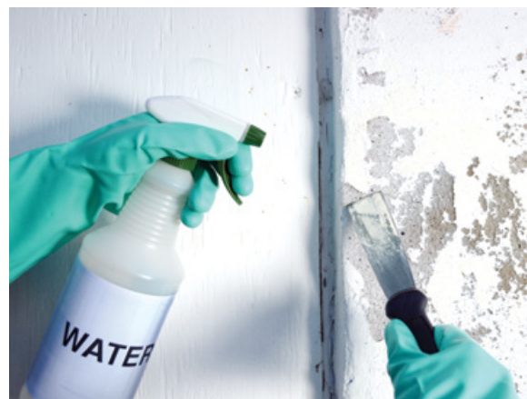
PHOTO: Wet-misting lead paint reduces dust hazard.
