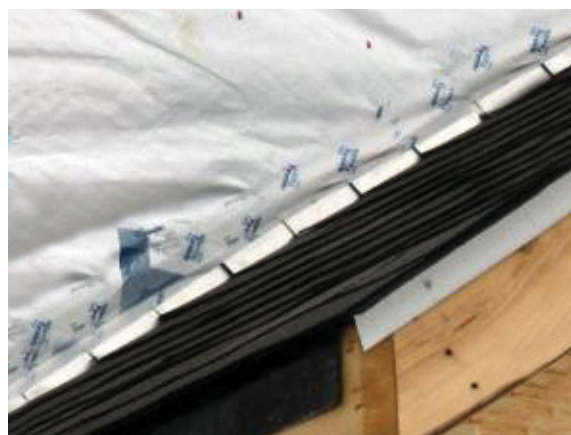
PHOTO: A water-resistant barrier layered over step flashing at a roof-to-wall intersection.
