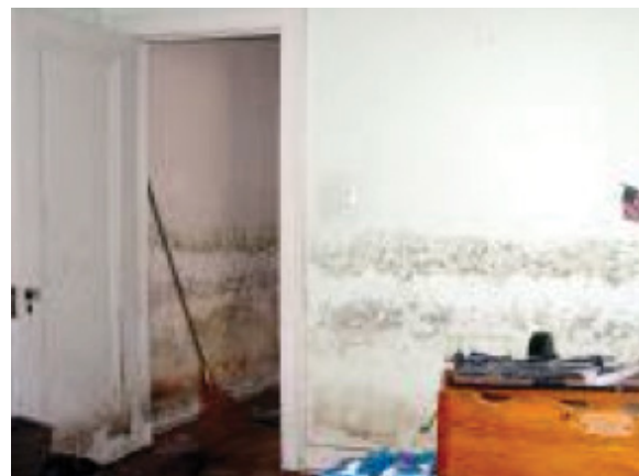
PHOTO: Mold growth in flooded home.
