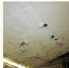
PHOTO 2: Ceiling damage resulting from roof leaks.
