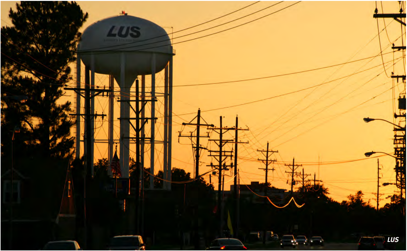
LUS managed water tower and power lines
