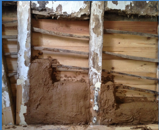
Bousillage infill hung on rungs between posts
